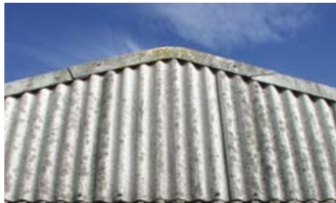
Asbestos cement wall cladding
